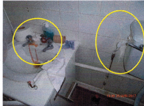
Photo 14: Outlets disconnected in the Kitchen toilet
