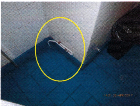
Photo 15: Deadend in Century house 1st floor Female toilet
