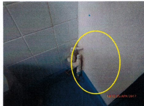
Photo 18: Deadend in Century house 1st floor Female toilet
