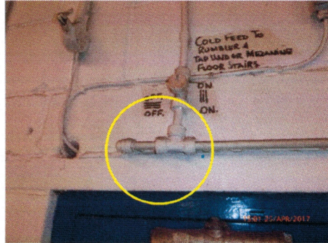
Photo 20: Deadend in Lada factory
