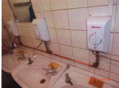
Photo 26: 3 water heaters in Lada workshop toilet that are connected and now redundant
